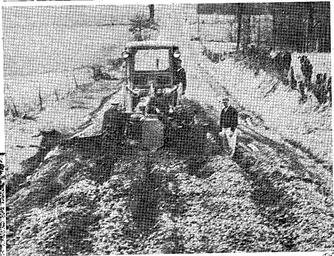
Shown above is the Washington township road maintainer mired in a mud hole on township road 205 just north of the Dave Thompson farm. When the picture was taken Tuesday, 14 loads of gravel had already been dumped in and the
